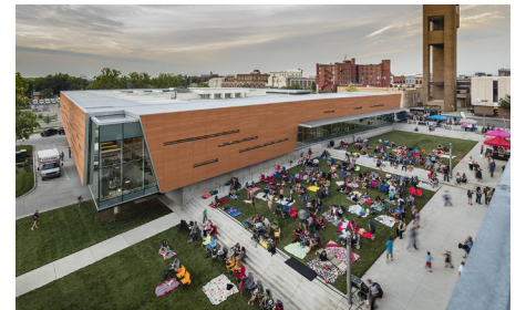
Aerial View of New Lawrence Public Library 1
